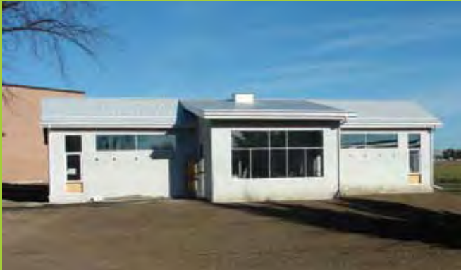
Minto Clifford Learning Centre under construction.
