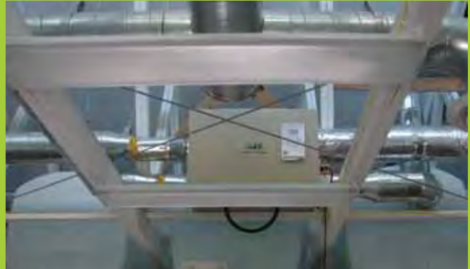
Rainwater Cistern located in the rafters, visible to students.
