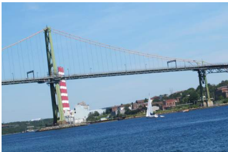
Below: The Angus L. McDonald Bridge, which joins Halifax to Dartmouth (top) and a Royal Canadian Navy ship in port (bottom).
